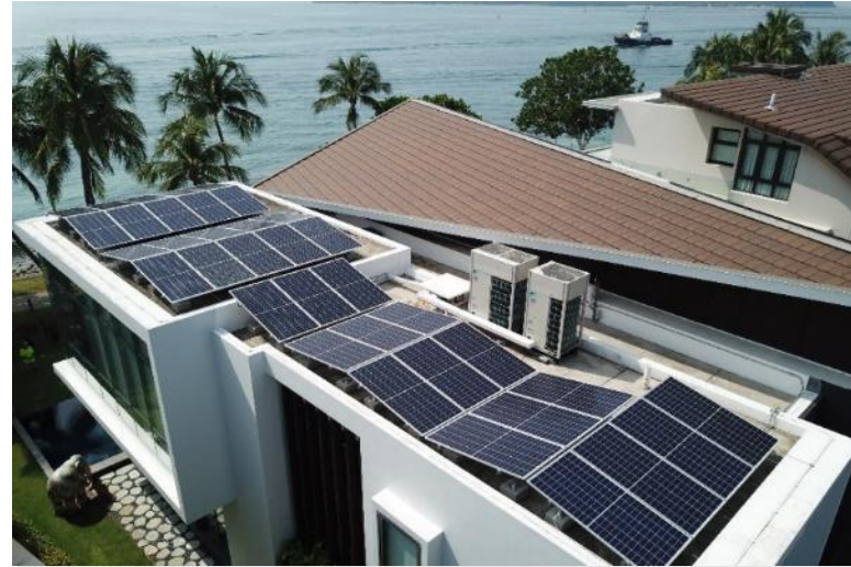
13kWp, Ocean Drive
