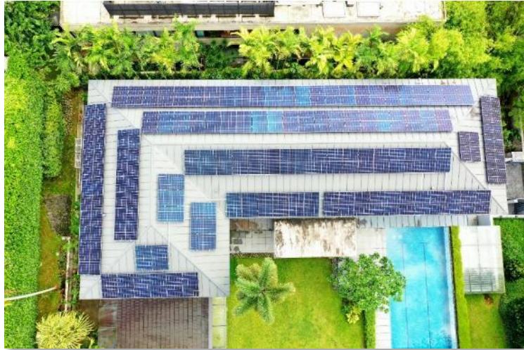
56kWp, Ewart Park
