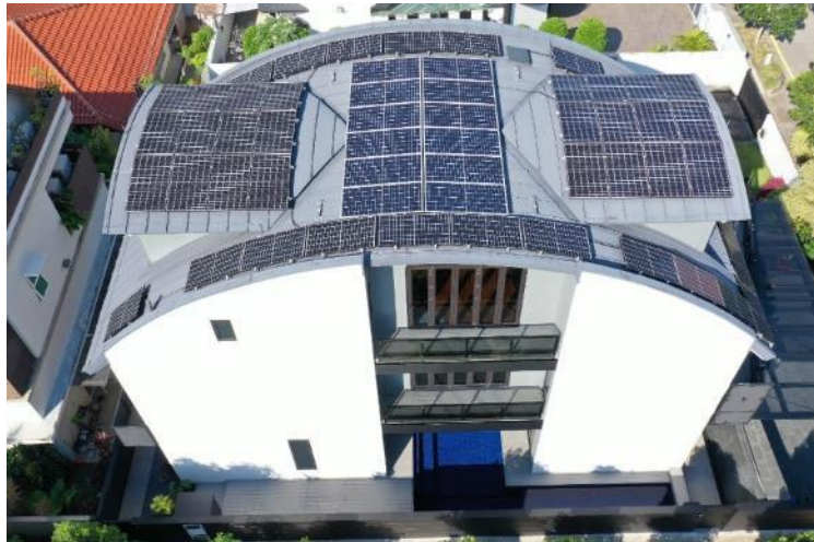
20kWp, Burnfoot Terrace
